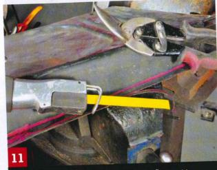
Cut away the excess metal including factory flanges. New flanges are needed so don't cut right back to the fold line
